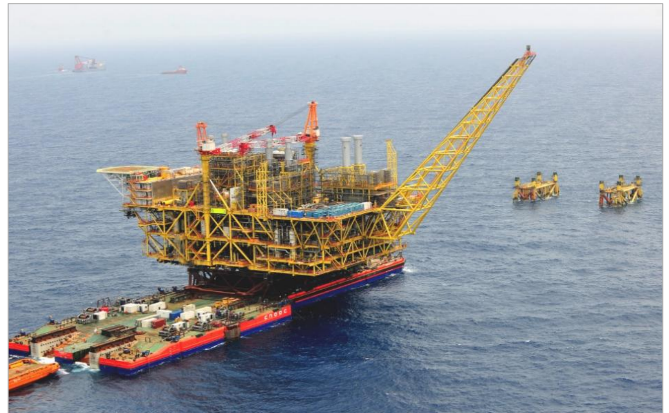
Topsides float over
