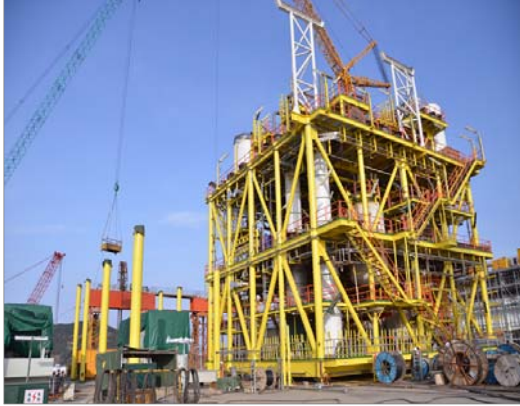
MEG pulled to position at +41 deck
