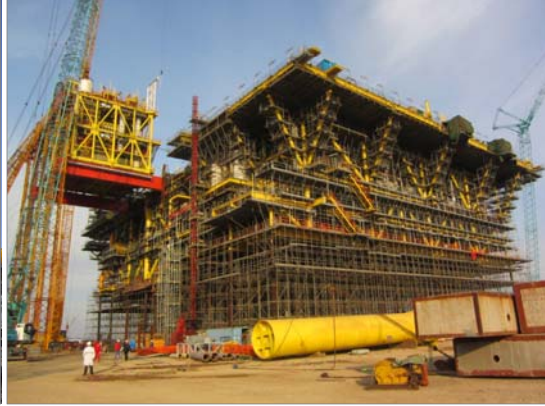
MEG jacked to +41 Level
