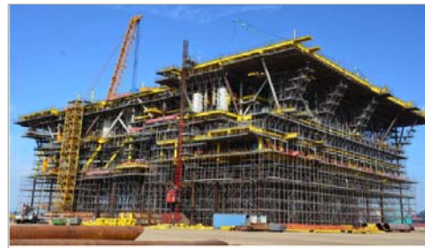
Topsides fabrication on schedule
